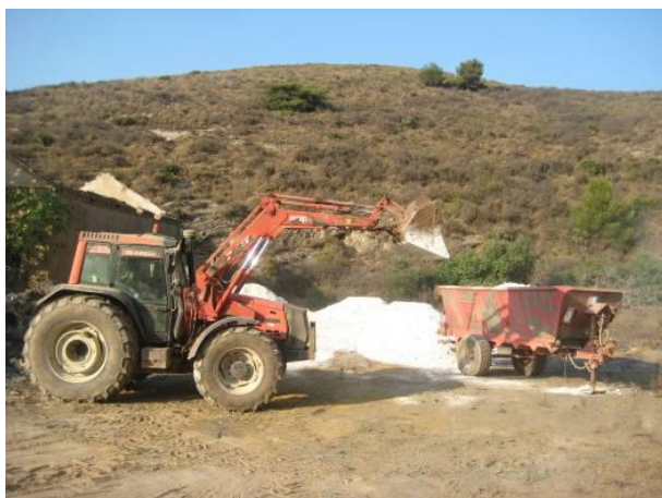
Figure 15 - Amendment application in Santa Antonieta mine tailing.
